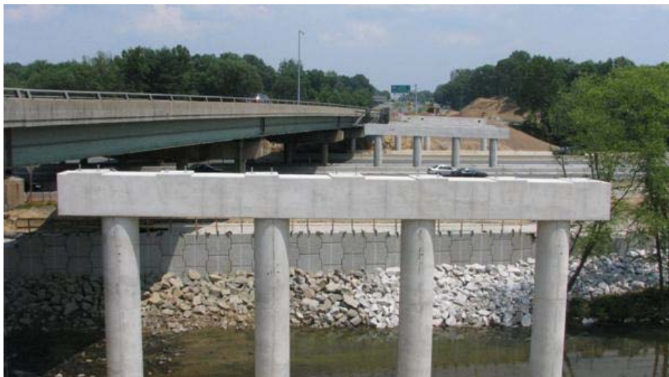
1 These bridge piers will support the steel beams.
